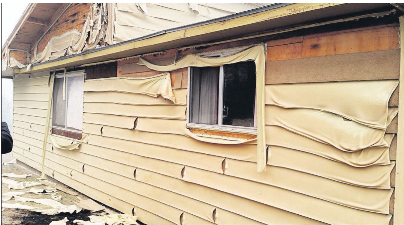
Siding has melted and fallen off, but Dortha Hoppe's house is still standing.
