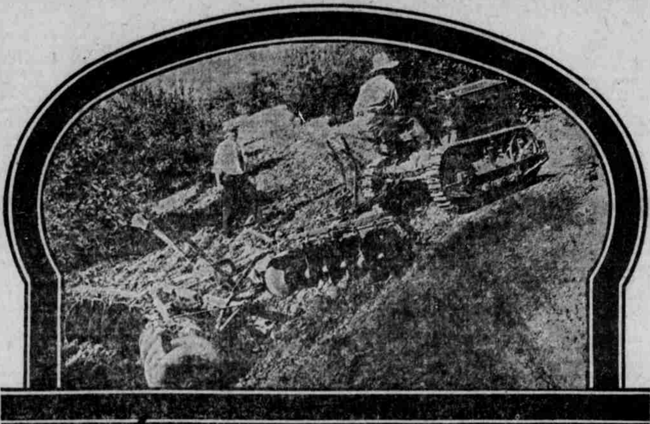
Cleveland Tractor with tandem disks working on 20 per cent grade
