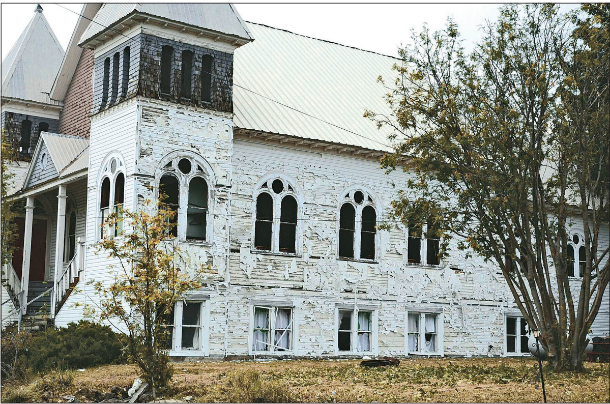
All the windows on the west side of the former United Methodist Church in Wallowa, many of them stained glass, were knocked out by a hail during a storm that passed through town Aug. 11. The siding, too, was seriously damaged.
