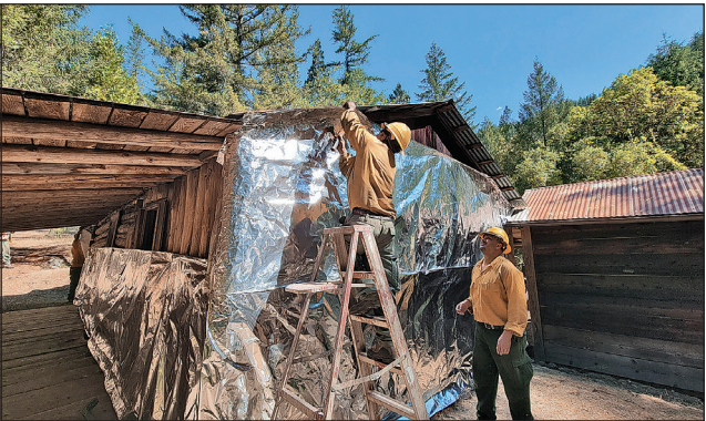
Fire crews structure-wrap the historic Whisky Creek Cabin on Aug. 23 with an aluminum fire blanket material designed to protect structures from sparks or embers and withstand intense heat from the Rum Creek Fire, the state's largest active fire. The cabin is one of the few remaining relics of the Rogue River gold rush era.
