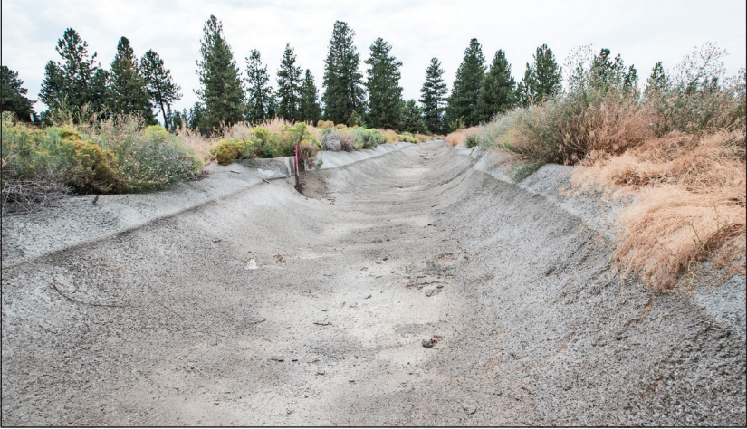
A small section of Arnold Irrigation District’s main canal lined with cement near Bend.
