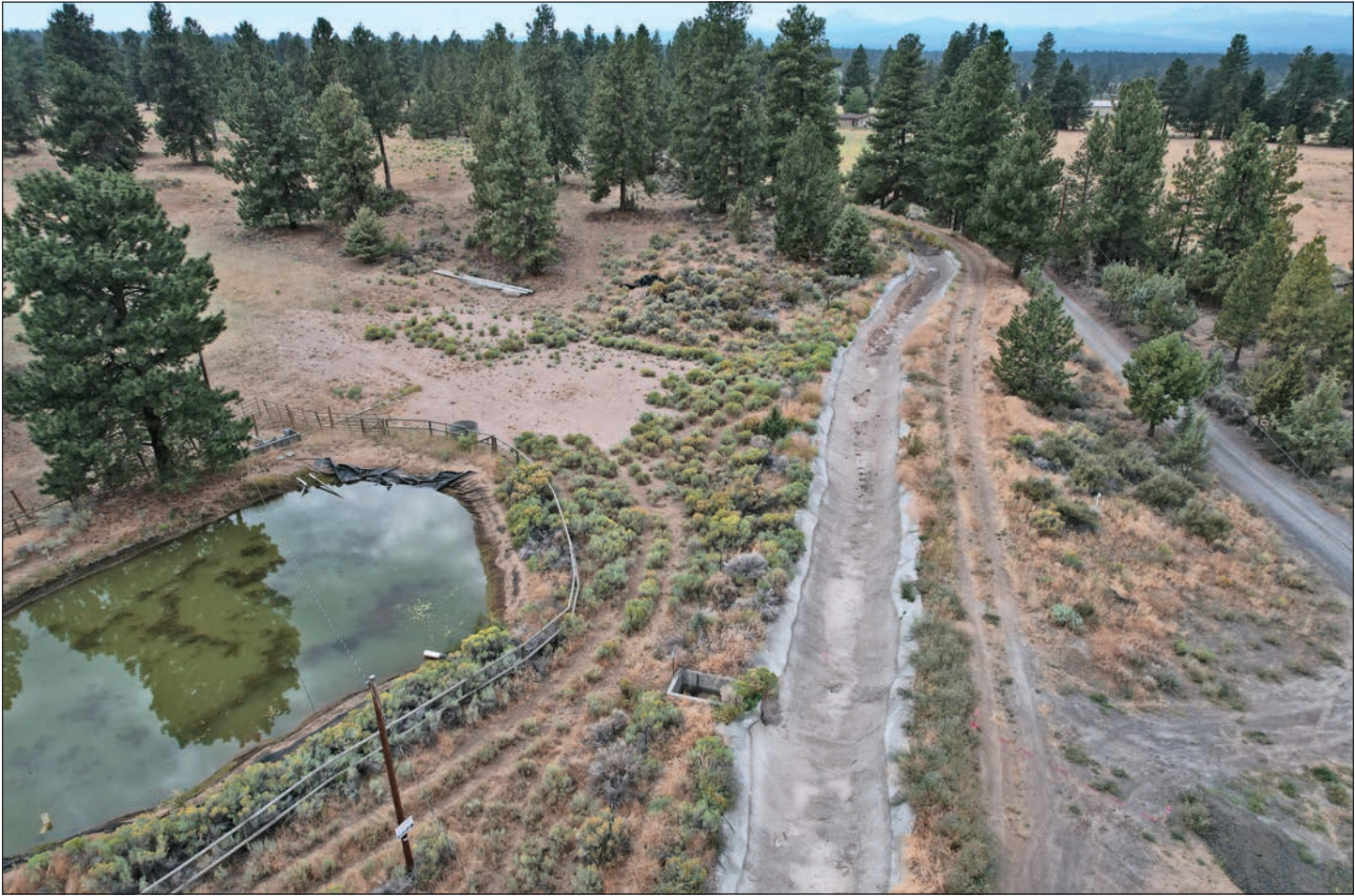
A small section of Arnold Irrigation District's main canal is lined with concrete near Bend.
