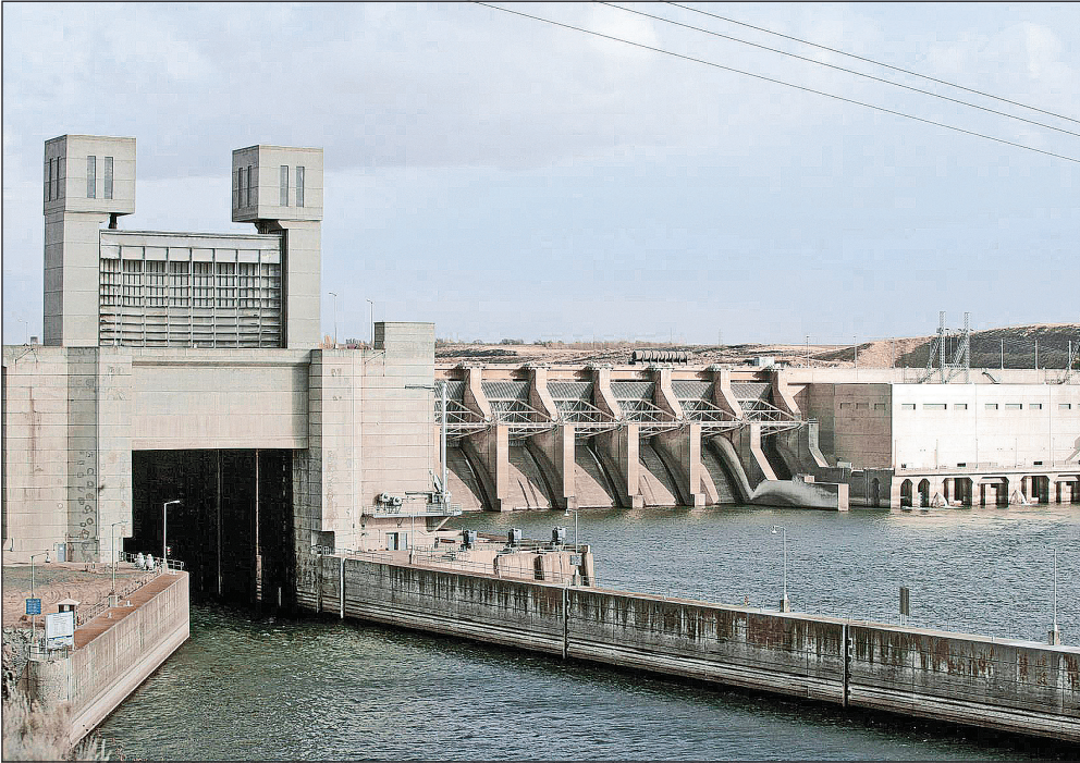
Ice Harbor Dam is one of four dams on the lower Snake River.
