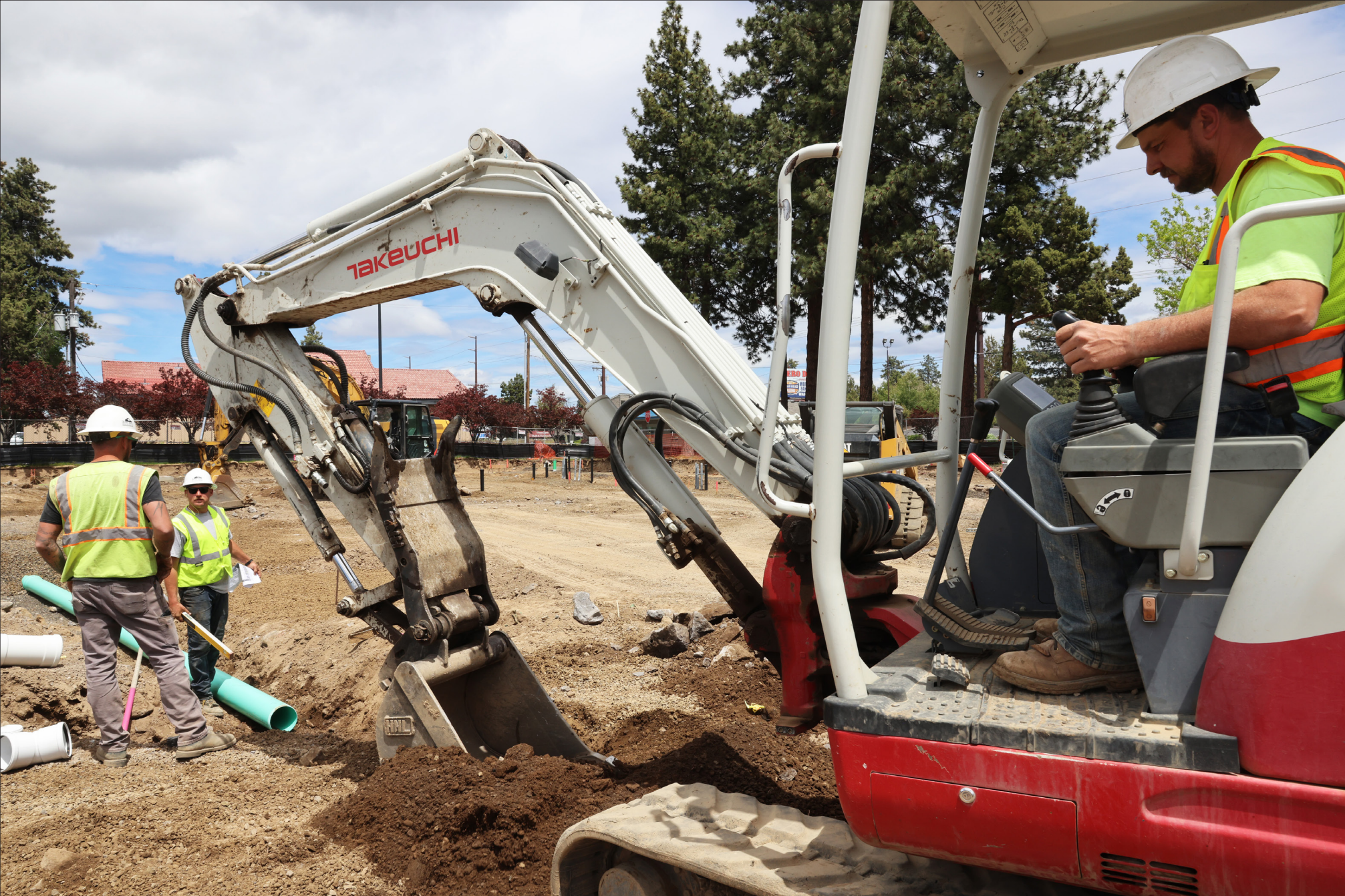
Chris Selby operates an excavator while working on the construction of a 6,040-square-foot, multiple-tenant building at Pinebrook Boulevard and Third Street in Bend.
