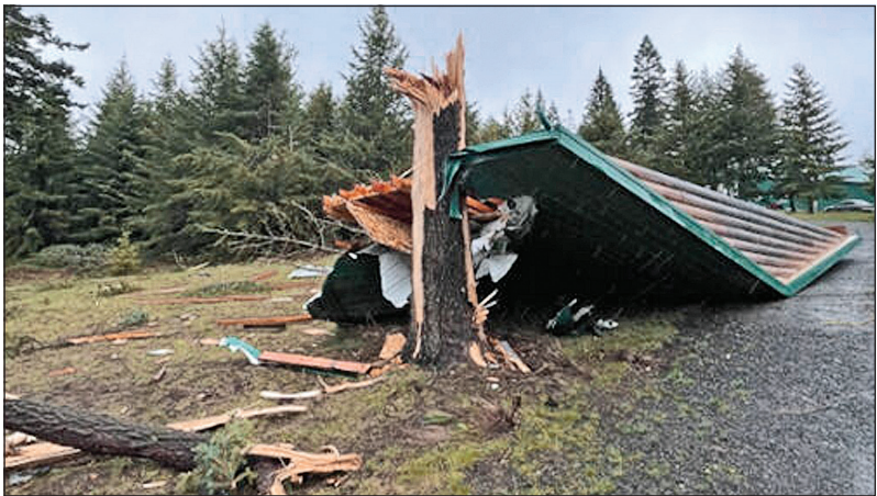
One of two tornadoes that touched down in Eastern Oregon on May 6 damaged buildings and uprooted trees.
