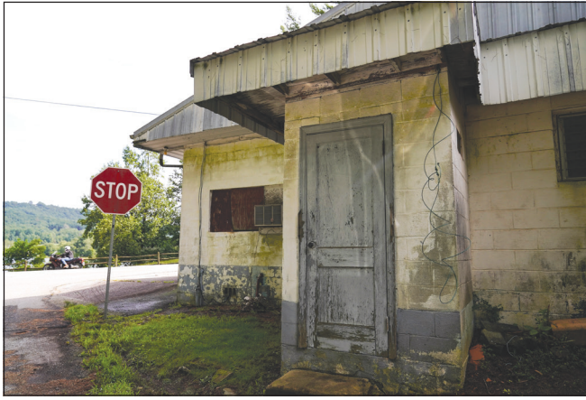
A building sits abandoned Thursday near Suches, Georgia. The Census Bureau has issued its most detailed portrait yet of how the U.S. has changed over the past decade.
