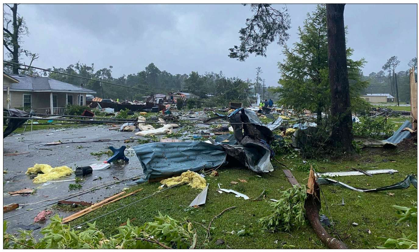
Debris covers the street in East Brewton, Alabama, on Saturday. Authorities in Alabama say a suspected tornado spurred by Tropical Storm Claudette demolished or badly damaged at least 50 homes in the small town just north of the Florida border.
