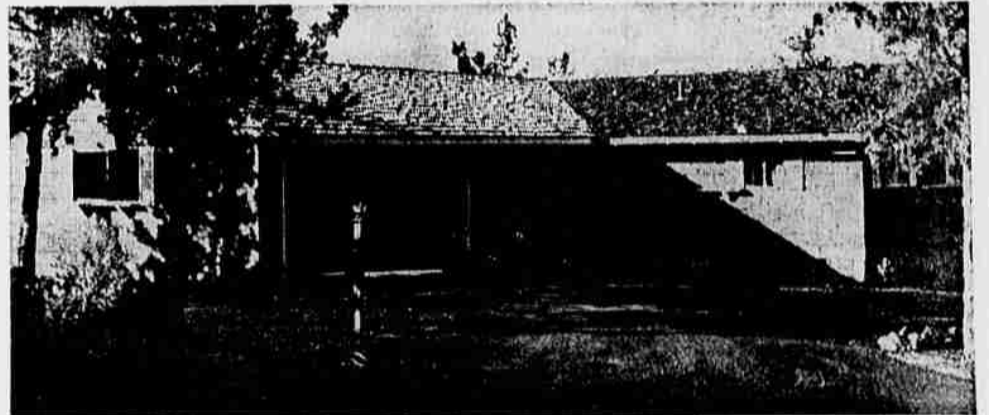
THIS IS THE HOME of Dr. and Mrs. Eugene Wegner at 1162 East Penn. This beautifully designed and constructed home features 3 large bedrooms, 2 baths, family room, living room with fireplace, country kitchen, double garage, split-shake roof, thermopane windows, separate entry hall plus a rustic siding that proves less costly in maintenance.
