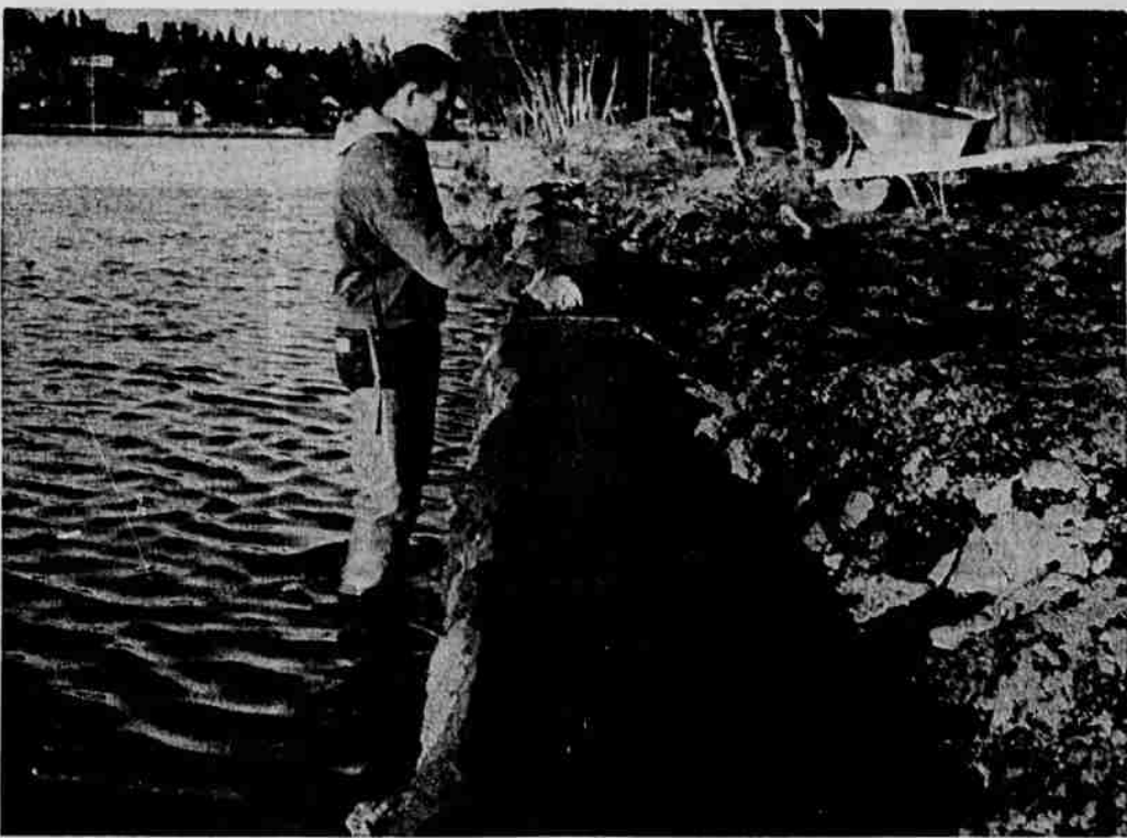
TAKING SHAPE—George Thompson of the Bend Park and Recreation Department works on 200 feet of rockwork on the east side of the Deschutes River in Drake Park. Fill behind the wall ends marshy spots and the wall will prevent trash from gathering along the river bank. Crews are working on the project as winter weather permits.
