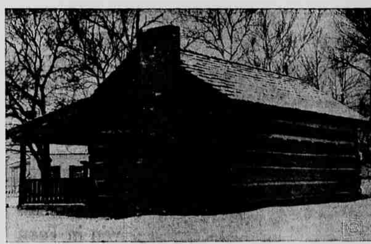
END OF ERA —Indiana's State Department of Education is closing all one-room schools by the end of the 1964 school year. Vincennes University, Vincennes, Ind., has erected this one-roomer on its campus for future generations of Hoosiers to visit. This ancient log cabin was enclosed within a barn for many years so its poplar logs are in a near perfect state of preservation. The interior will be restored to the style of the early century.
