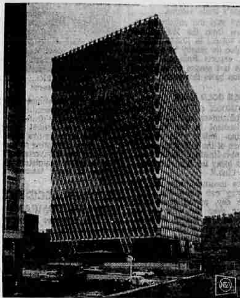
INSIDE-OUT BUILDING — One of the most unusual buildings going up in Pittsburgh, Pa., in its "renaissance" development called Gateway Center, is the new IBM building pictured above. The honeycombed exterior is actually the building's structural steel framework. The outside shell is constructed of four giant trusses, one for each side. Each truss rests on two concrete pillars. A vertical core in the center of the building adds additional support and is the only interior column.
