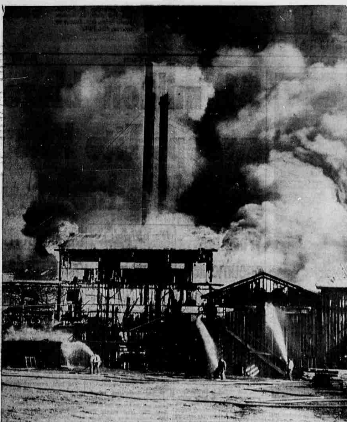
TITE KNOT PINE MILL CRUMBLES IN FIRE — Wind-swept flames Wednesday afternoon about 4:30 o'clock destroyed the Tite Knot Pine Mill in Redmond, with the loss set at a million dollars. It was one of Central Oregon's most costly mill fires. Tall smoke stacks are shown here outlined against a great cloud of smoke that rolled up from the mill as the fire swept through the mill, only recently modernized. Reconstruction will start as soon as possible. This picture was taken by Bulletin photographer Nate Bull minutes after smoke started billowing up from the pine plant.
