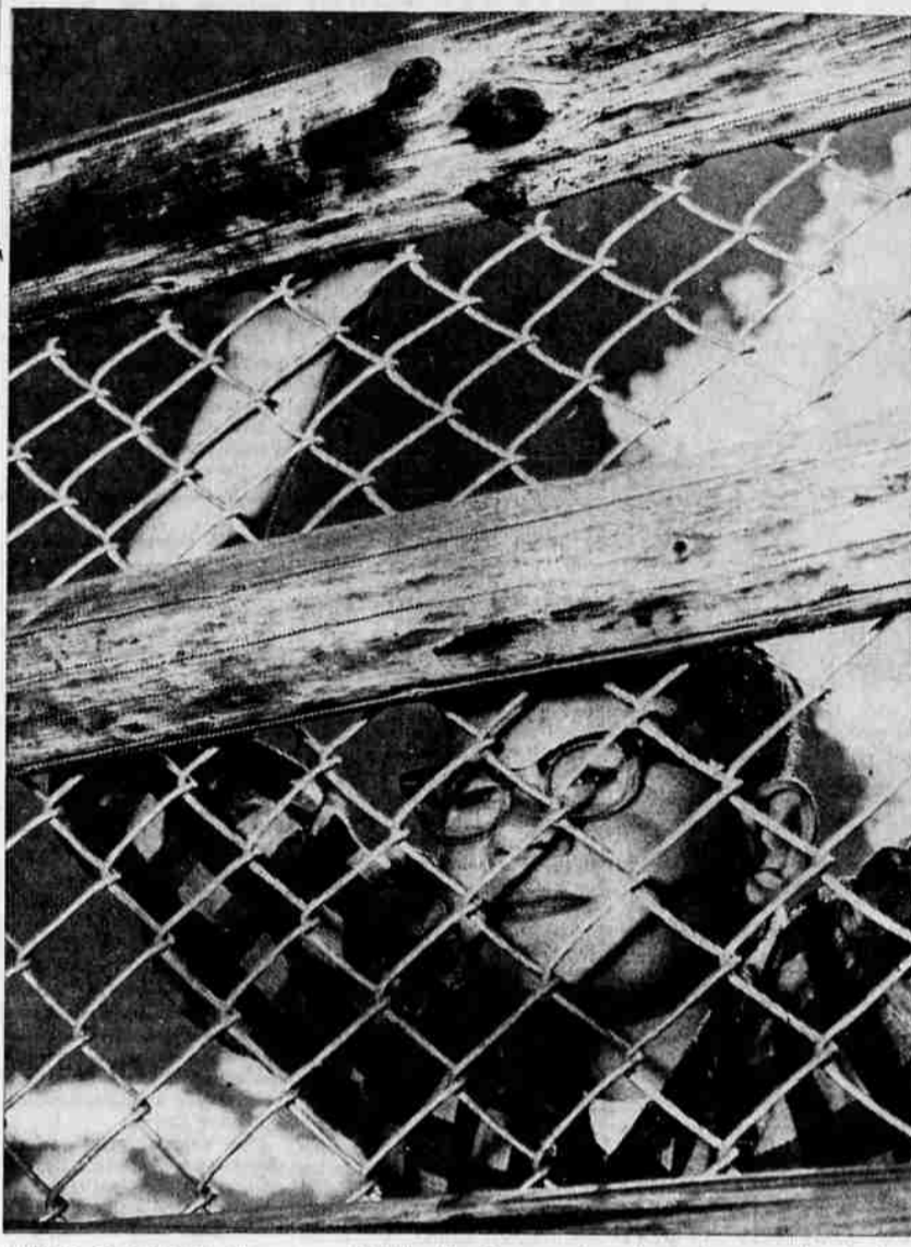
SHIELD OF SAFETY—Eleven-year-old Mike Marvin peers through sturdy woven-wire fencing fastened last week to rails of Drake Park footbridge. Protective fence will prevent tots from slipping through rails and tumbling into treacherous river. Another fence is soon to be installed at Gilchrist footbridge, from which two youngsters tumbled to their deaths this past year.
