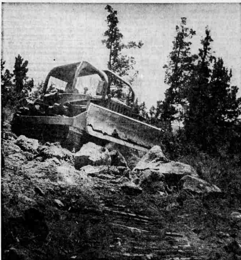
TOUGH 'DOZING FACED —First work under the contract between the C.O.C. board and Steinlicht Construction Company was started Monday on the college grounds just west of Bend. Work on an access road is pictured here. Leonard Moe has this subcontract.
