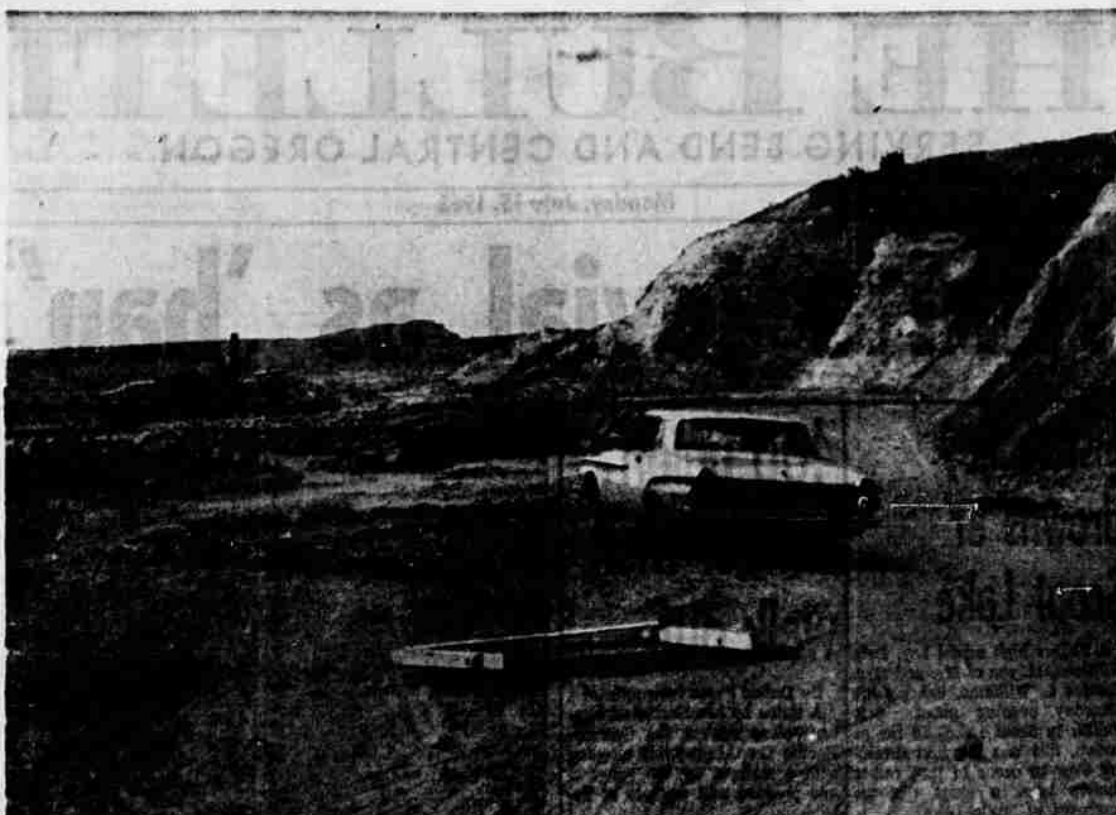
FACE OF HILL SLIPS, SHIFTS HIGHWAY — A huge chunk of a steep hill near Clarno on the John Day River is slipping these days, carrying a section of the Antelope-Clarno road with it. A highway crew is attempting to cut a new grade into the hill above the slippage zone. The section is still on the move, with deep cracks appearing in the construction area overnight. (Photo by Phil F. Brogan).
