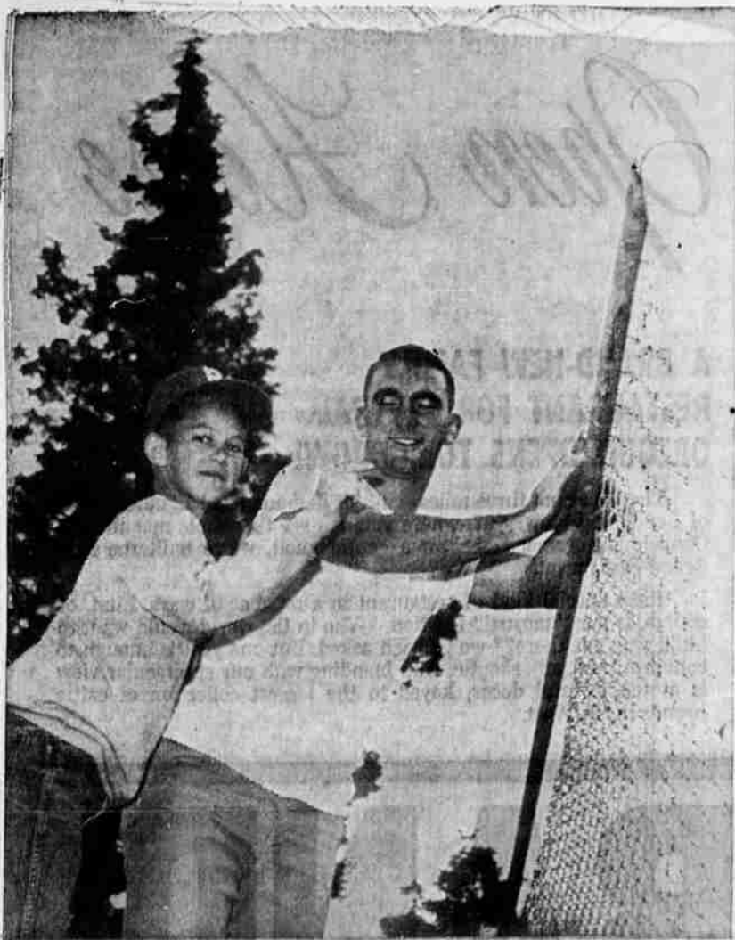
BACKSTOP INSTALLED—Andy Cole, 10-year-old Brandis Bantam Leaguer, is shown giving a few pointers to city employee Wally Donohue on the construction of a backstop on Kingston Field. The installation of the backstop, financed by the Little League and erected by the recreation department, will enable American Bantam League games and practices to be held on the field.
