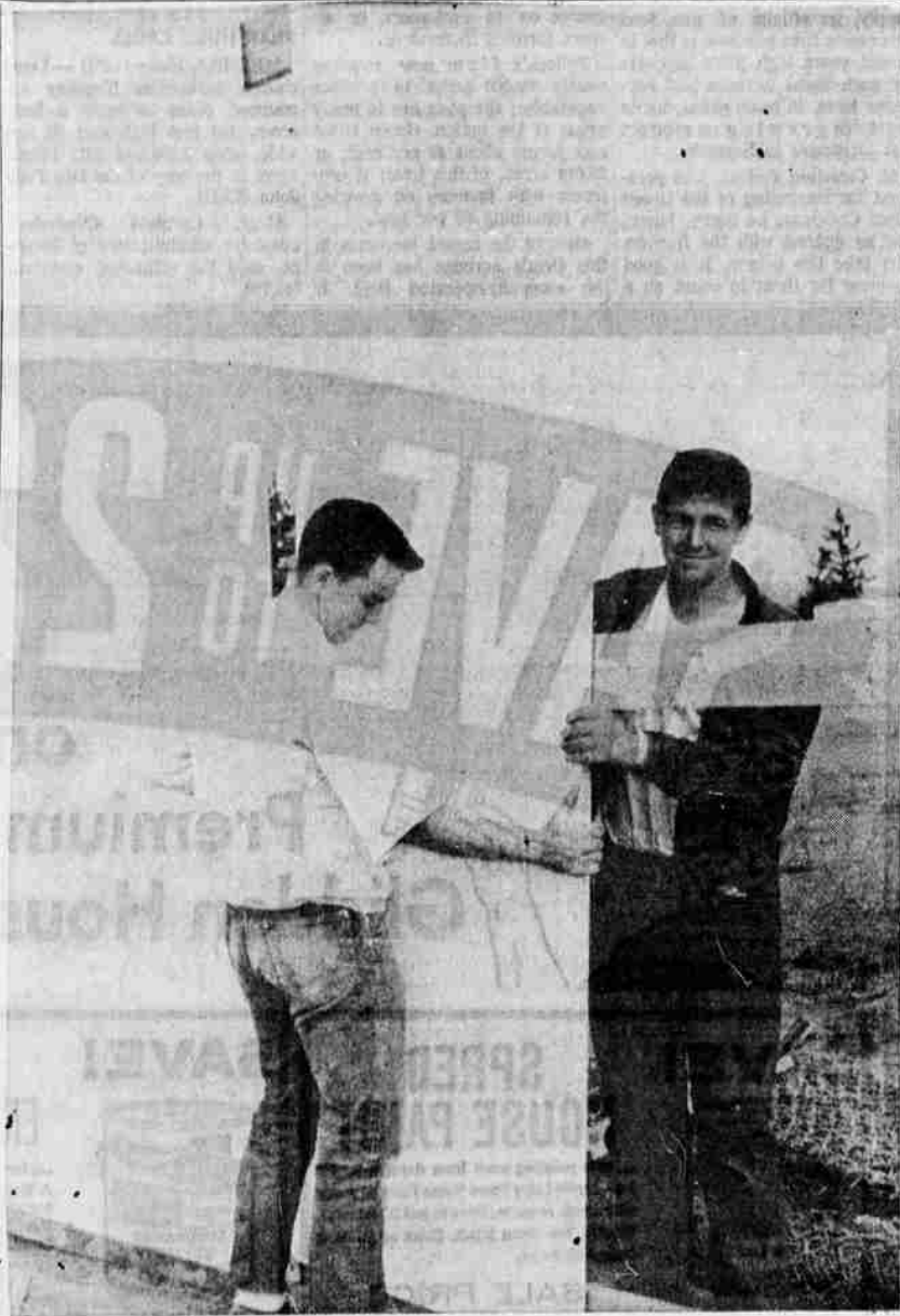
FENCE BUILDERS—City employees Benny Hamilton and Les Bryan are shown putting sheet metal panels in place on the new Bend Municipal Ball Park fence. Construction of the new fence began last year, with the entire old fence slated for replacement. The new fence has extended all outfield distances by about 30 feet. Work being done above is on the south side of the field, with only the east fence remaining to be replaced.
