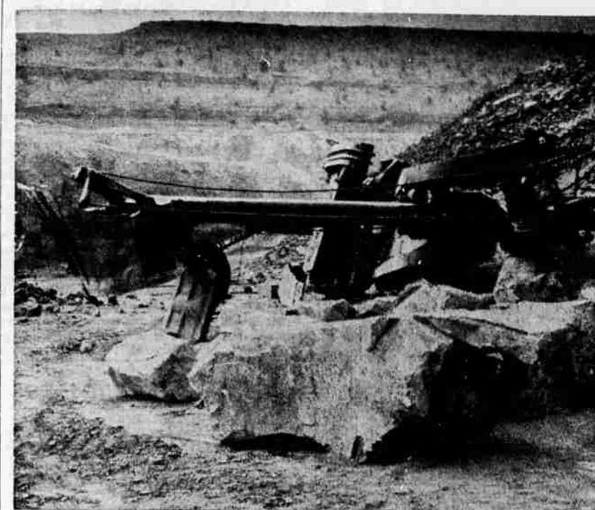
JUNKED — A $250,000 power shovel, its boom twisted and housing smashed, went over a 125-foot embankment, in a mechanical failure Friday at Round Butte Dam. Three men were riding the shovel but jumped clear; one is hospitalized with fractures, in Prineville.
