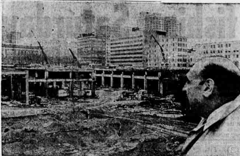
DREAM COMING TRUE — Big hole for big project, Cleveland's new underground exhibition hall, is viewed by a fellow who knows all about its beginnings — Anthony J. Celebrezze, Cleveland's mayor before becoming health, education and welfare secretary in President Kennedy's cabinet.
