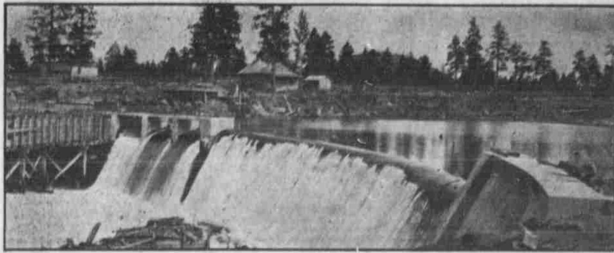
NORTH CANAL DAM WHICH COMPANY ASKS STATE TO TAKE OVER, AND COMPLETE THE SYSTEM.
