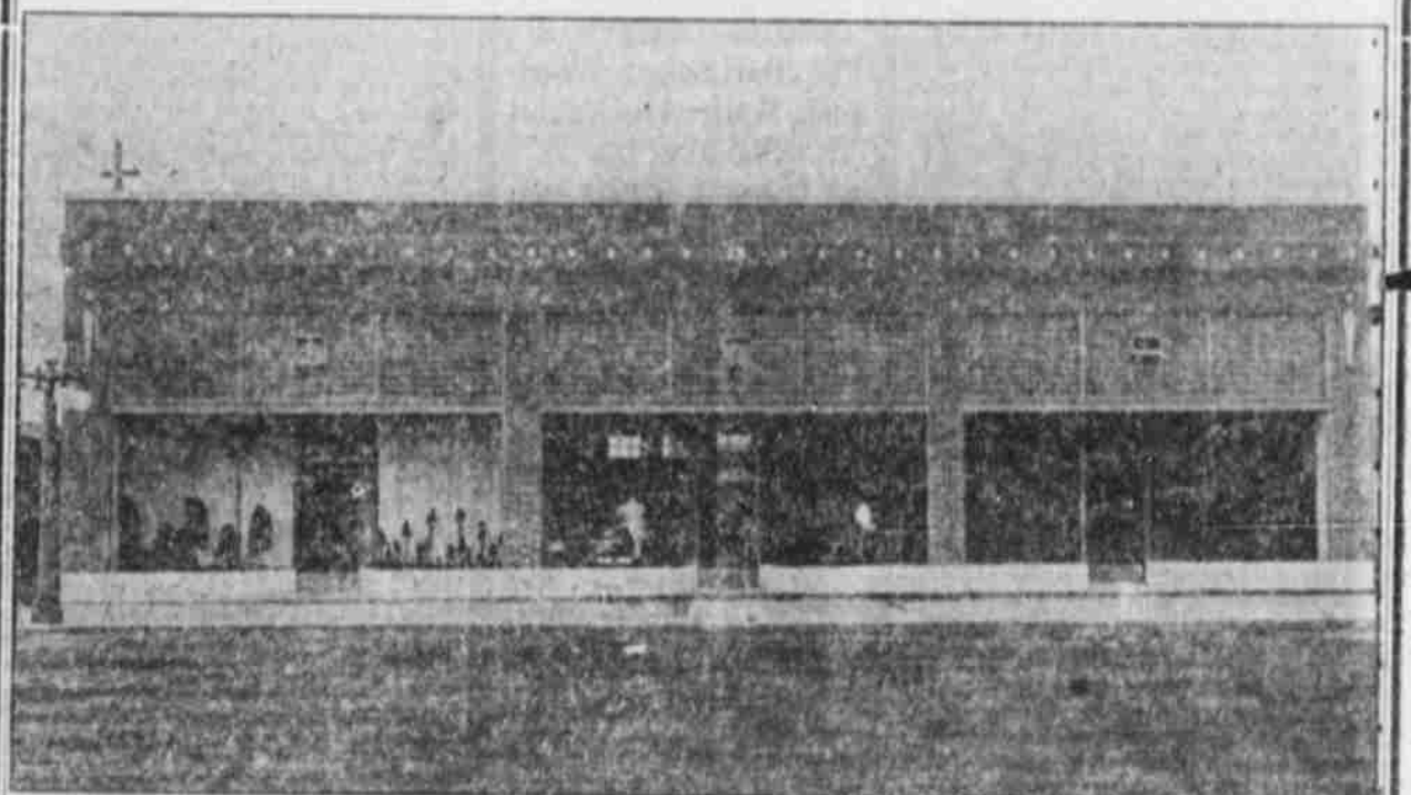
Erected at a cost of nearly $10,000, by R. B. Mutzig, this is one of the best business buildings in Bend. The front is of imported brick and the other walls of locally manufactured brick. It contains three store rooms occupied by A. L. French's clothing store, Innes, Davidson & Bartlett's barber shop and between Bond and Wall streets. Each store room contains a basement at the rear. Mr. French and Innes, Davidson & Bartlett have hot air heating plants, and the latter firm also has tub and shower bath facilities. The space below the plate glass front of the building is tiled, and a cement sidewalk and cluster lights add to the attractiveness of the building.
