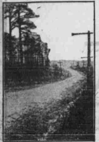
A CURVED ROAD IS TRULY A POOR ONE. It is used as a foundation with a three or four inch covering of granite also rolled and watered.
