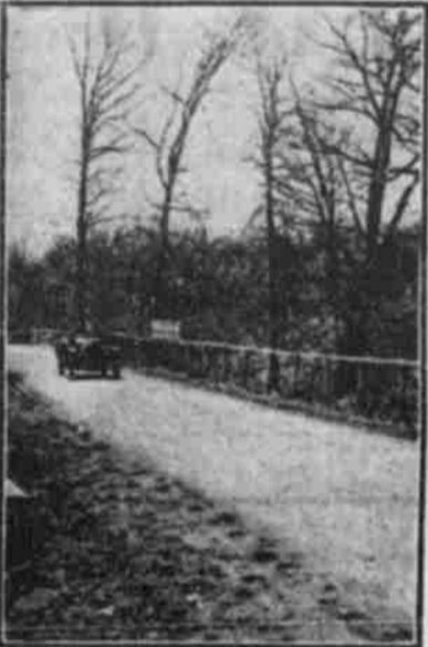
A STATE HIGHWAY IN MARYLAND.
