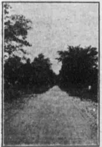
MACADAM ROAD IN NEW JERSEY.
