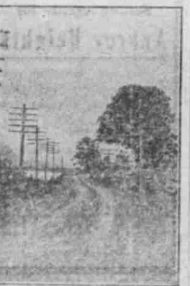
WATER BOUND MACADAM ROAD IN NEW HAMPSHIRE.
