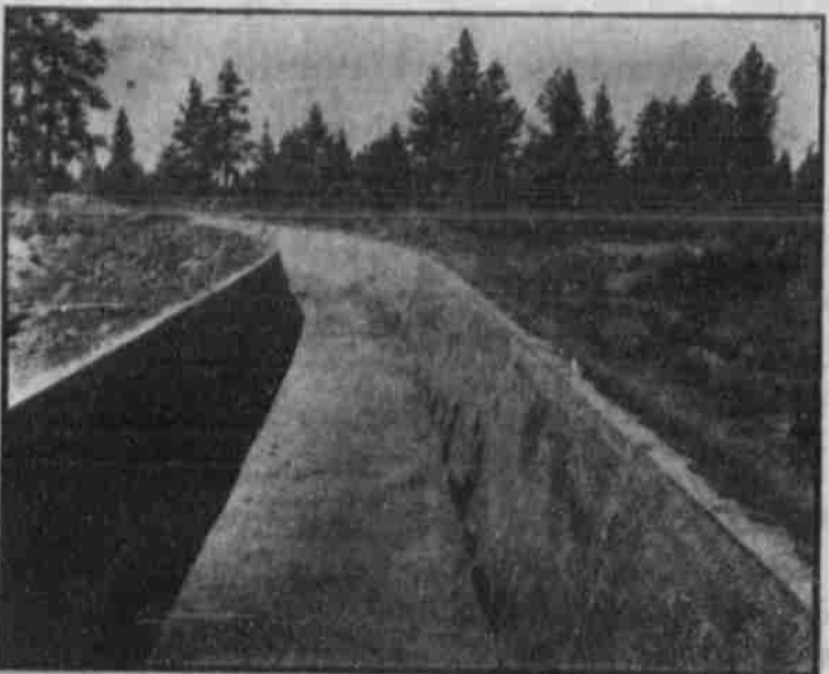
"North Canal" Concrete Lined Flume
