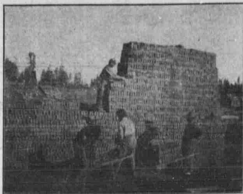
PILING THE FIRST KILN OF BRICK FOR BURNING, TWO MILES WEST OF BEND,
