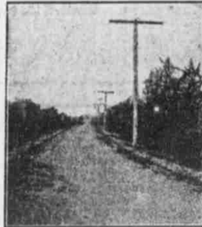
A GRAVEL ROAD.
