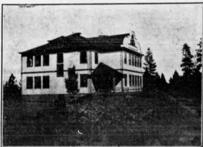
BEND'S PUBLIC SCHOOL BUILDING.
