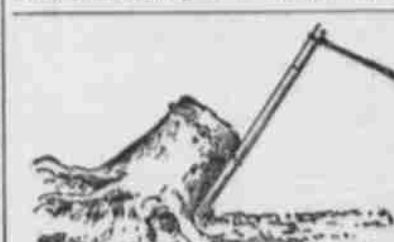
FOR PULLING THE STUMPS.
