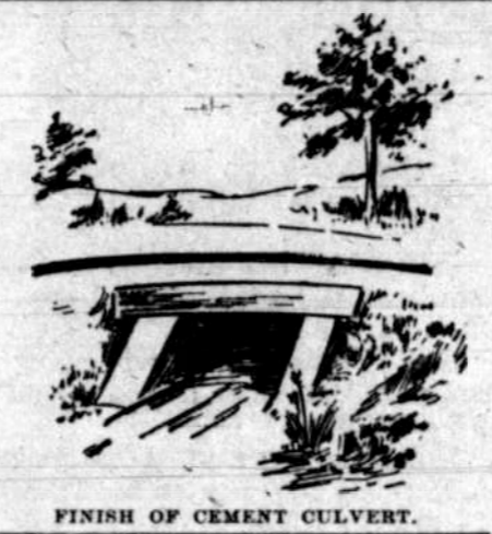
FINISH OF CEMENT CULVERT.
