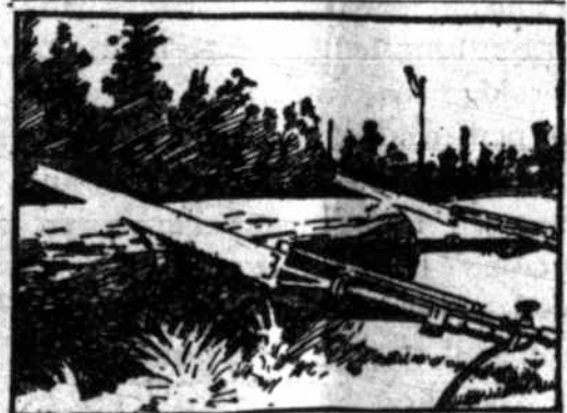
SAWING WITH COMPRESSED AIR.
