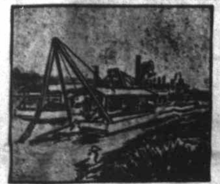
DREDGES IN THE CANAL.
