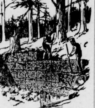
HISTORIC WALL UNCOVERED.
