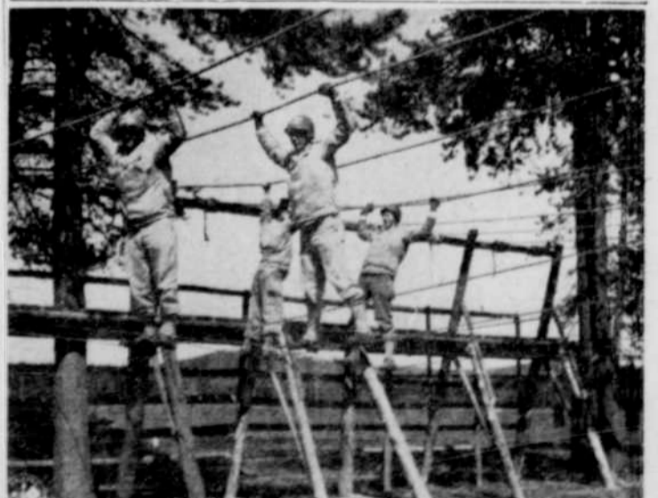
Post Signal Photo Lab. The Corps of Engineers quickly adopts—and improves—any idea of merit. The above method of crossing a stream has been used by Pacific island natives for centuries. Lines are thrown over tree limbs, and the free ends regained with the aid of a long pole. This training device, erected under the supervision of Lt. Warren L. Meyer of Camp Abbot, assists men in becoming sure-footed and confident in precarious situations.
