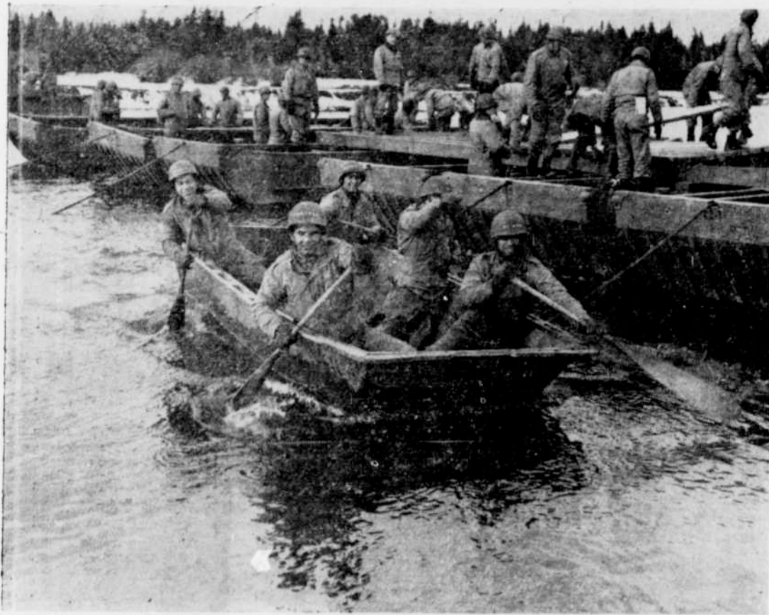
In all theaters of operations, the Corps of Engineers prepares the way for the advance over land and water. It builds roads and bridges of several types. Above photograph shows Camp Abbot Army Service Forces engineer trainees learning by doing. They are laying a heavy ponton bridge across the Deschutes river in record time.
