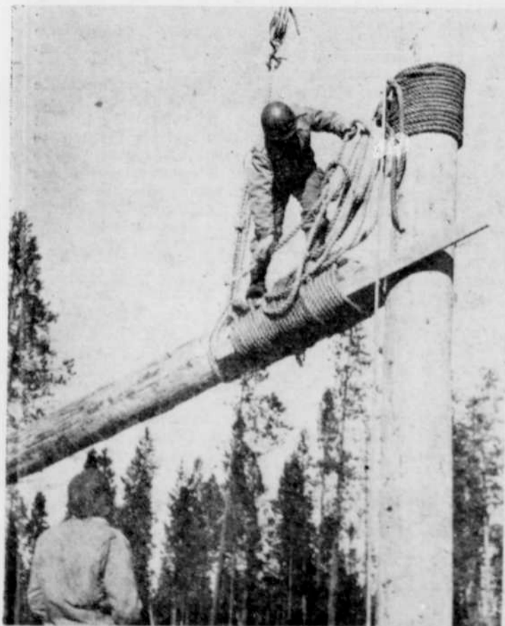
The above picture shows one phase of the rigging application course, an important part of combat engineer training. The trainee's current problem is to apply correctly his knowledge of the "square knot."
