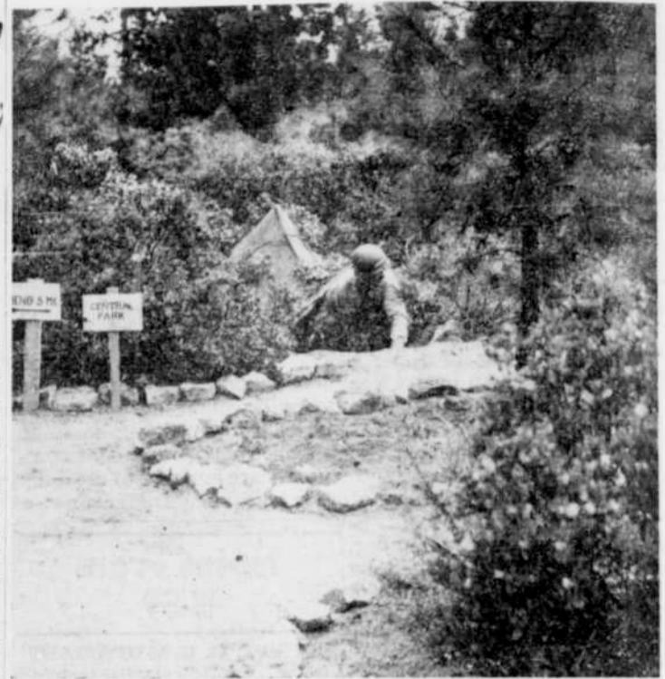
A bit of Gotham in the Oregon woods north of Camp Abbot. Corps of Engineers trainees of 51st battalion, utilizing local plant life, designed garden spot and named it "Central Park," as sign at right of man emerging from foxhole shows. —Photo by Signal Corps Photo Lab.
