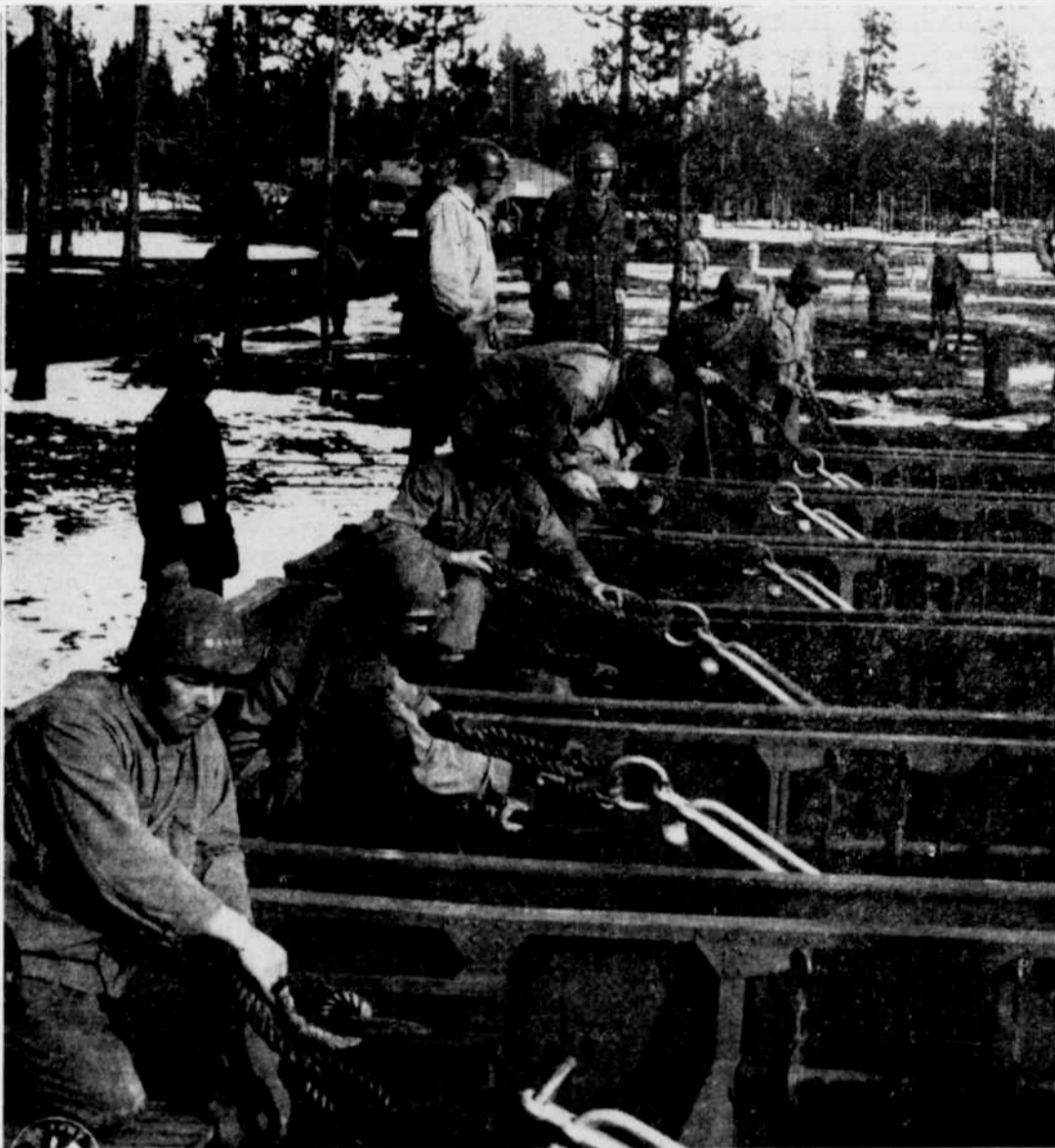
Learning to tie anchor hitches, sheet bends, mooring hitches, timber hitches, square knots and bowlines is a small but important phase of combat engineer training—important because an engineer's life sometimes depends on the security of a knot. Photo shows the first station of the Rigging Application course. Here, trainees are tying anchor hitches. The entire course is composed of five stations, through which the trainee travels hoisting himself to the tops of towers, climbing rope ladders, making lines secure in a multitude of ways. At the finish he slides down a high line from a 20 foot tower while sitting in a bowline on a bight.
