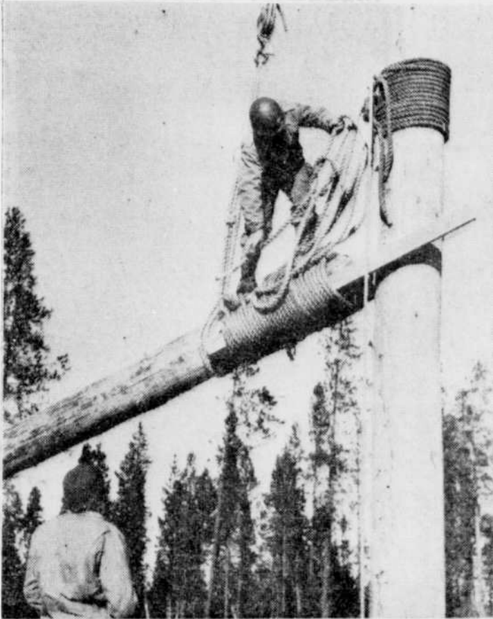
The days of ship and sail are recalled in this photograph of an Engineer trainee undergoing one phase of training in rigging at Camp Abbot. The trainee's current problem is that of correctly applying his knowledge of the "square knot."
