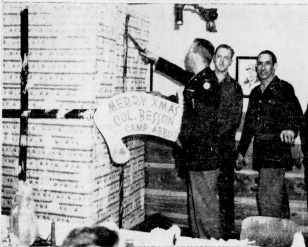
Col. Frank S. Besson, ERTC commander, is shown welding a bayonet to open what probably was one of the largest Christmas presents in the United States. The package concealed the doorway to the new addition to the Officers' Mess and marked the formal opening of the new structure Christmas Eve. Holding the bayonet sheath is Warrant Officer Marvin L. Tragerman.
