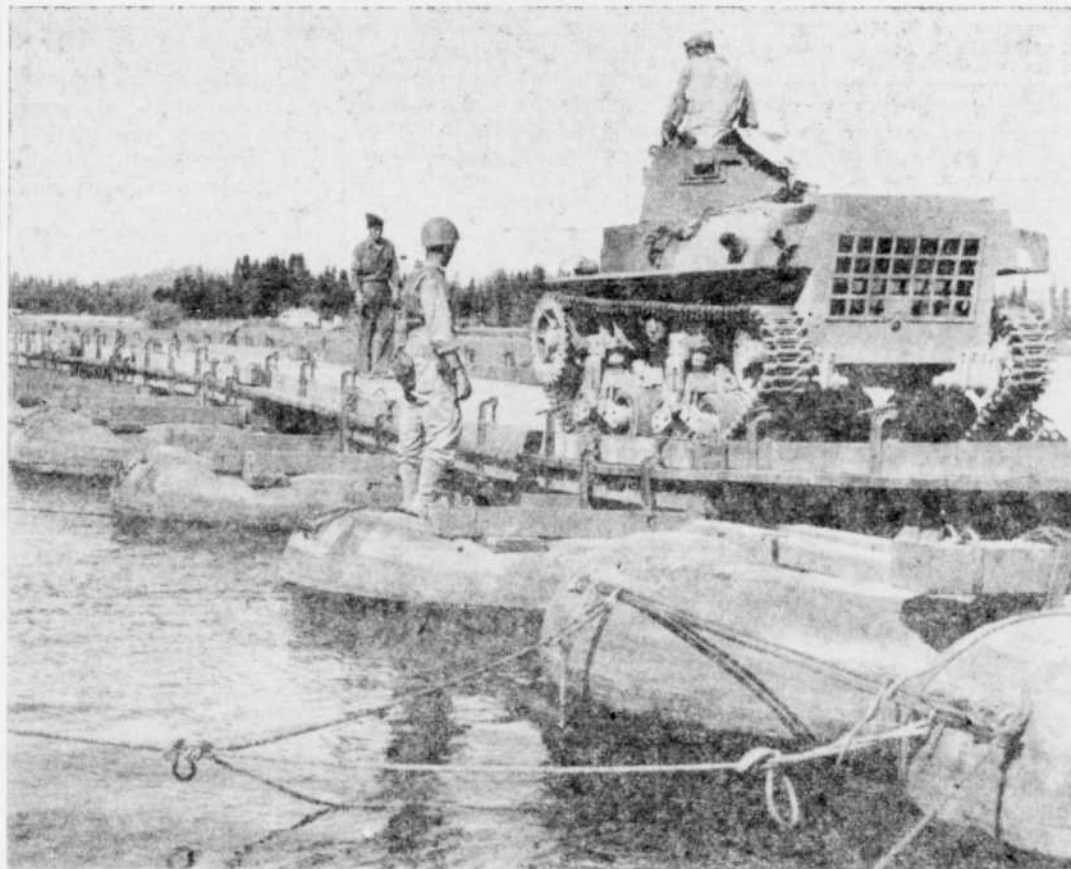
A light tank is shown testing a pneumatic ponton bridge constructed by soldiers of the Engineer Replacement Training Center on the Deschutes River here. Easier to construct than the metal type span, the pneumatic bridge can be assembled in far less time than the older model, is easier to transport and can be entirely submerged and still remain buoyant. An example of the army's conservation program: Salvage materials from other type ponton bridges are used as balk and chess.
