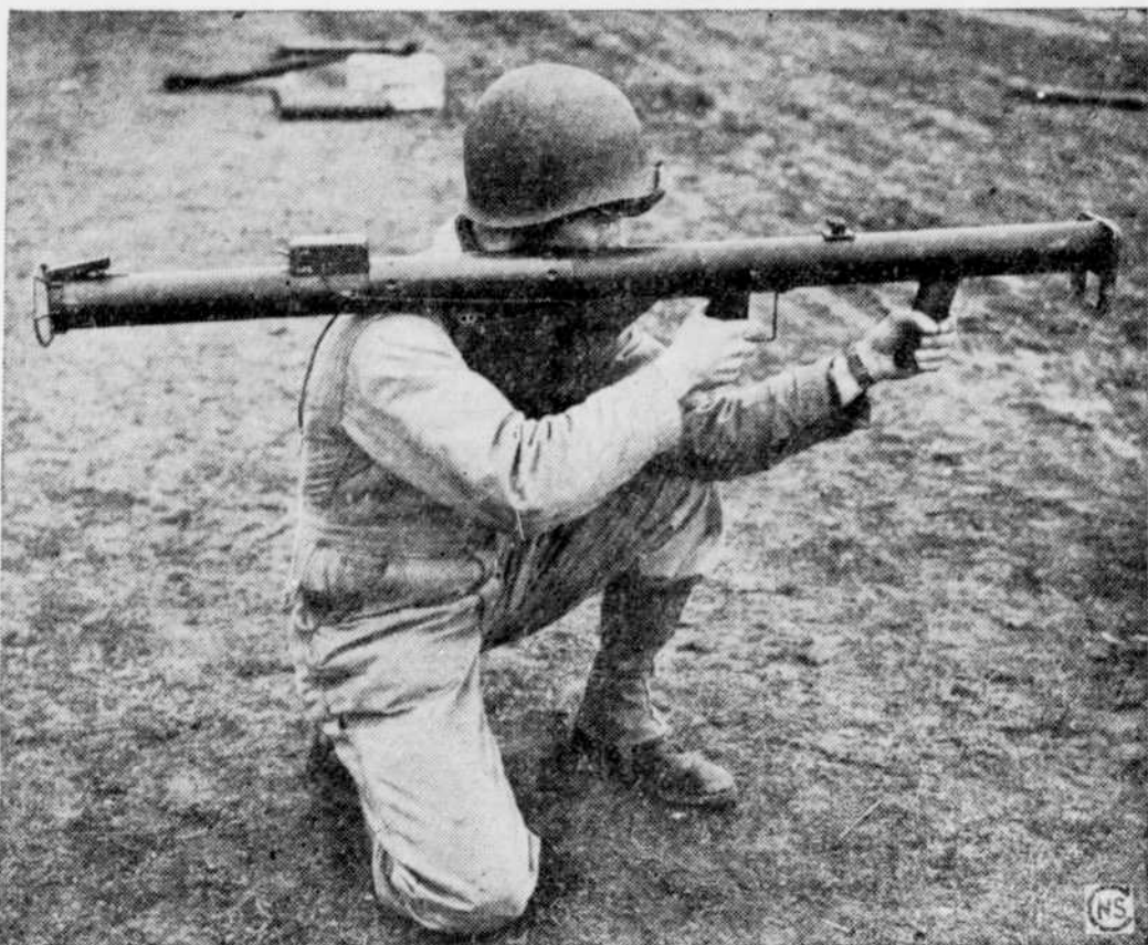
Bazooka is the slang name for this weapon which has proved so deadly against enemy tanks and which has been classified "secret" until recently. It's GI name is Launcher, AT, M-1. It can be operated by one man in a pinch and shoots a big spurt of flame out its tail. The guy who holds it feels practically no kick at all.
