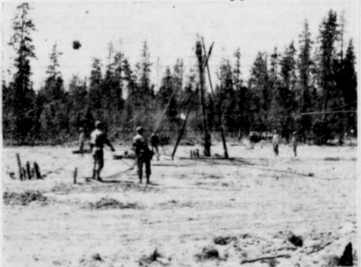
ABBOT ROOKIES LEARN HOW TO MOVE HEAVY LOADS— All soldier-engineers must acquire the technique of rigging—expedient methods of moving bulky loads. Shown above are recruits of the second platoon, D-51, constructing a gin pole, which, when completed is a standardized means for loading and unloading heavy equipment, placing heavy bridge timbers and other uses taught in the ERTC. (ENGINEER Photo by Hahn.)
