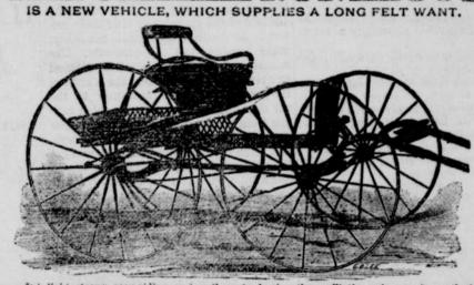
It is light, strong, easy riding, and well made, having three elliptic springs underneath the refuses springs are made especially for this wagon and will carry 500 kes, with ease), double it, shed axles, the best steel tire, leather dash, and a solid beared bottom. It has a box it he seat for small packages, and a wire guard around the back for holding larger packages, lead for catalogue and prices. Manufactured by GARDINER & CROSS, Louisville, Ky.
