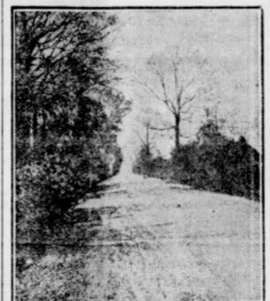
A CONCRETE ROAD.
