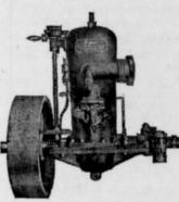
represent a distinct step in advance in marine engina construction. No outside water pipes, not an ounce of superfluous weight, all bearings adjustable to take up wear.
